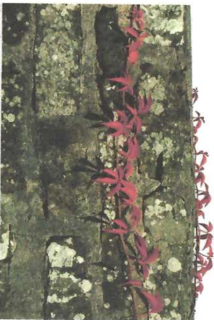
No coping - just a skim of modern cement replaces the original topping.
