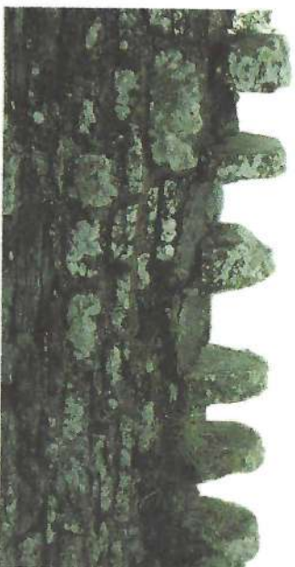
Half-round tooled coping stones unusually widely spaced, perhaps indicating that some have been removed prior to modern repair.
